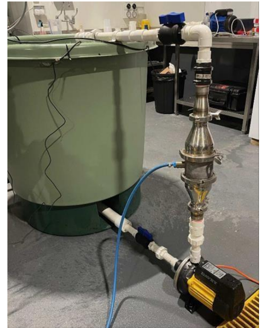
500 L tank setup with NB injector
