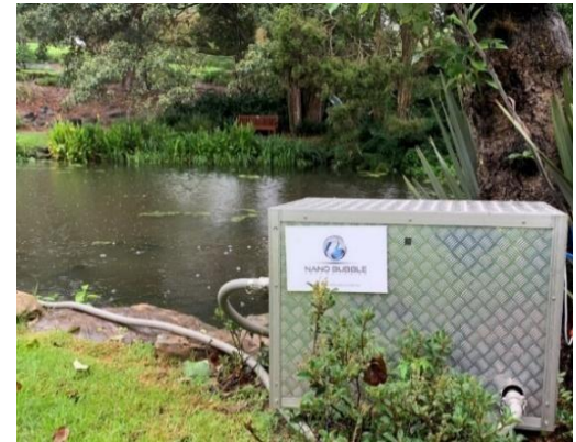
Photo 1: 3-Cell NBT injector installed for water treatment
